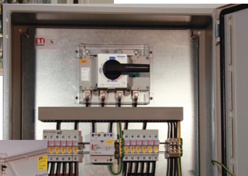
DC junction box (CH gPV fuses)
