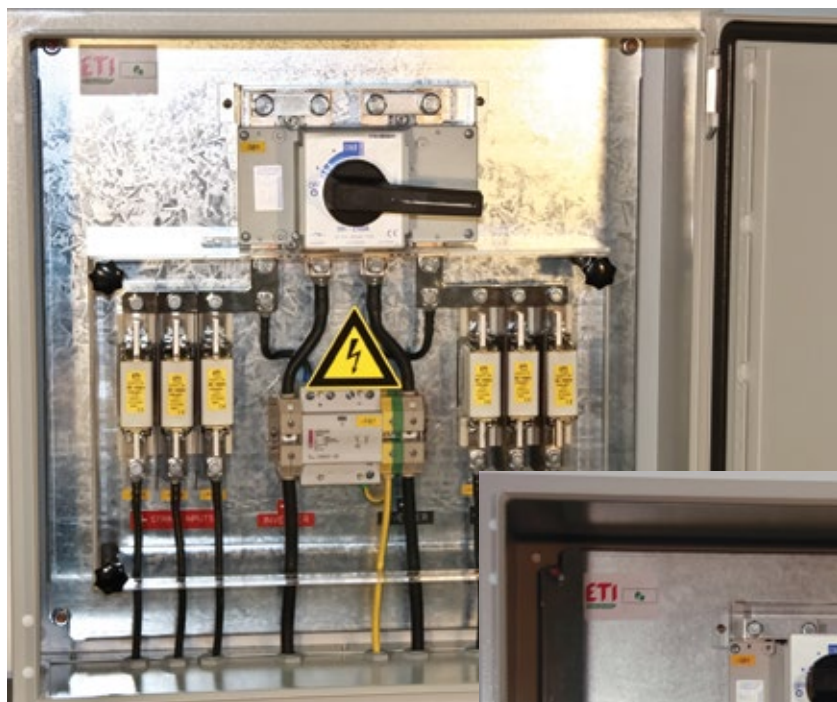
DC junction box (NH gPV fuses)
